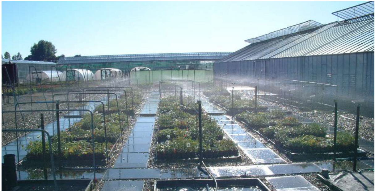
Fig P23 Overhead sprinkler irrigation in use 19/06/01
